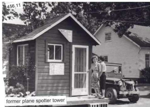
Norton Hill tower—now renovated
