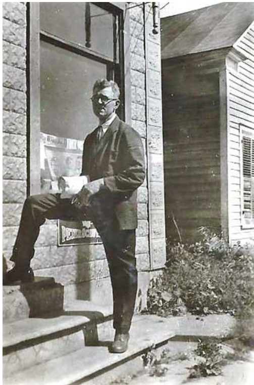
Tentatively identified as Bill "the Barber" Neidlinger; building on east Main Street
