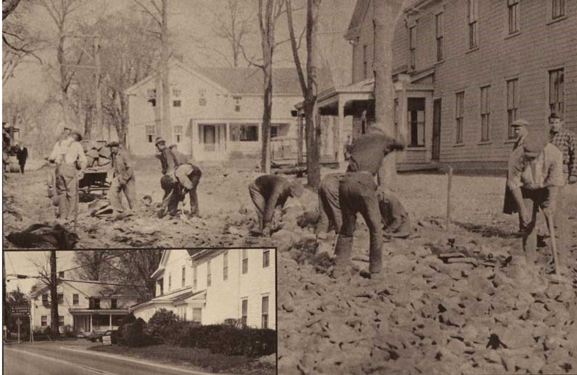
April 1992: The advent of the paved road made automobile travel much easier, but the making of such a road was back-breaking work. These men are pounding creek rock endwise into the dirt, thus making for a solid base in the later 1920s. The road from Cairo-Freehold-Greenville, pictured here at Freehold's four corners, would eventually eclipse the east-west road, today's County Route 67, as Freehold's main road. The building on the right was Parks Inn, today the Freehold Country Inn. The house to the left was the Lacy house and is still owned by Janet Lacy Halstead. (courtesy of Janet Halstead)
