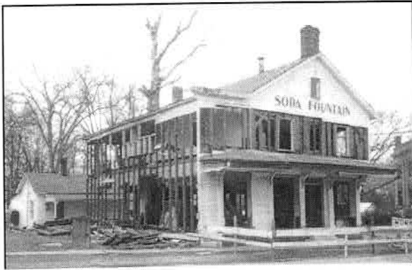
Razing of Corner Restaurant - early 1960s
