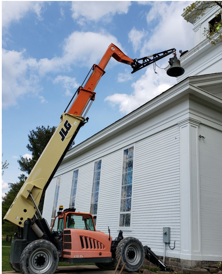
Removal of bell in 2021
