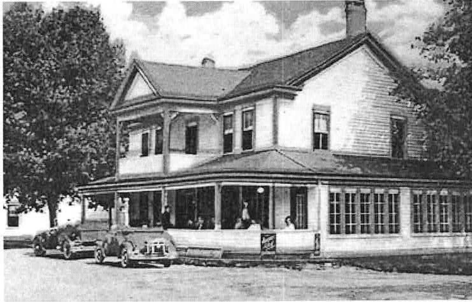
Freehold Inn (Parks', Freehold Country Inn, etc.) The tall front columns of today not yet built
