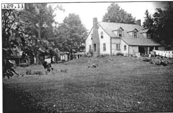
Talmage-Atwater-Baumann House View from south, rear
