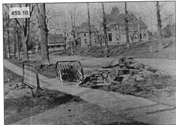
View from the upper school driveway, to Powell house and beyond
