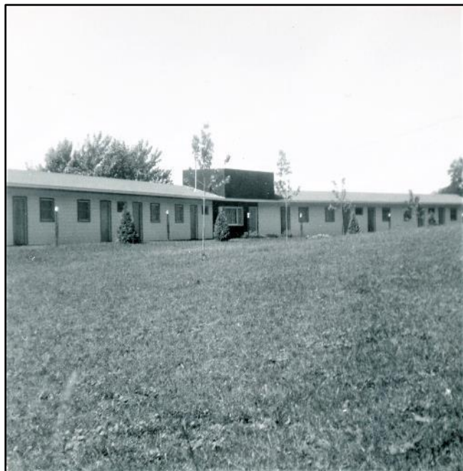
Model "B" view from the south. The "darker" center structure is the TV Room.
