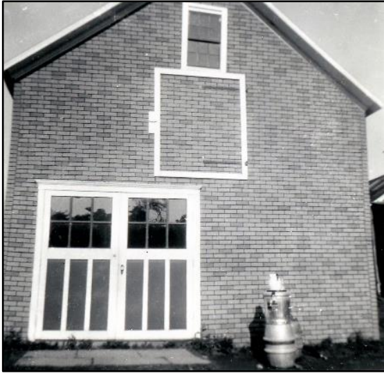
The front of the original Recreation Hall with the "morning after" remanent of the Beer Keg.
