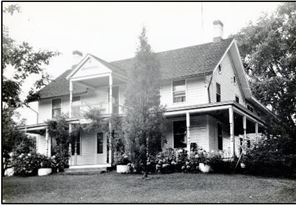
Another front view of the Original Main House.
