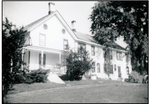
East side of the Original Main House. (The New Dining Room will be added here)
