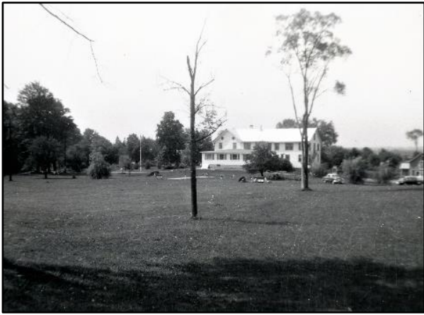
The Dining Room addition can be seen as viewed from the north.
