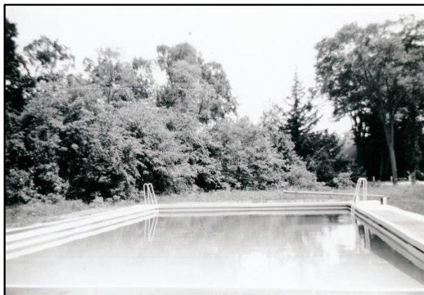
The Pool looking from "Shallow End" towards the "Deep End"
